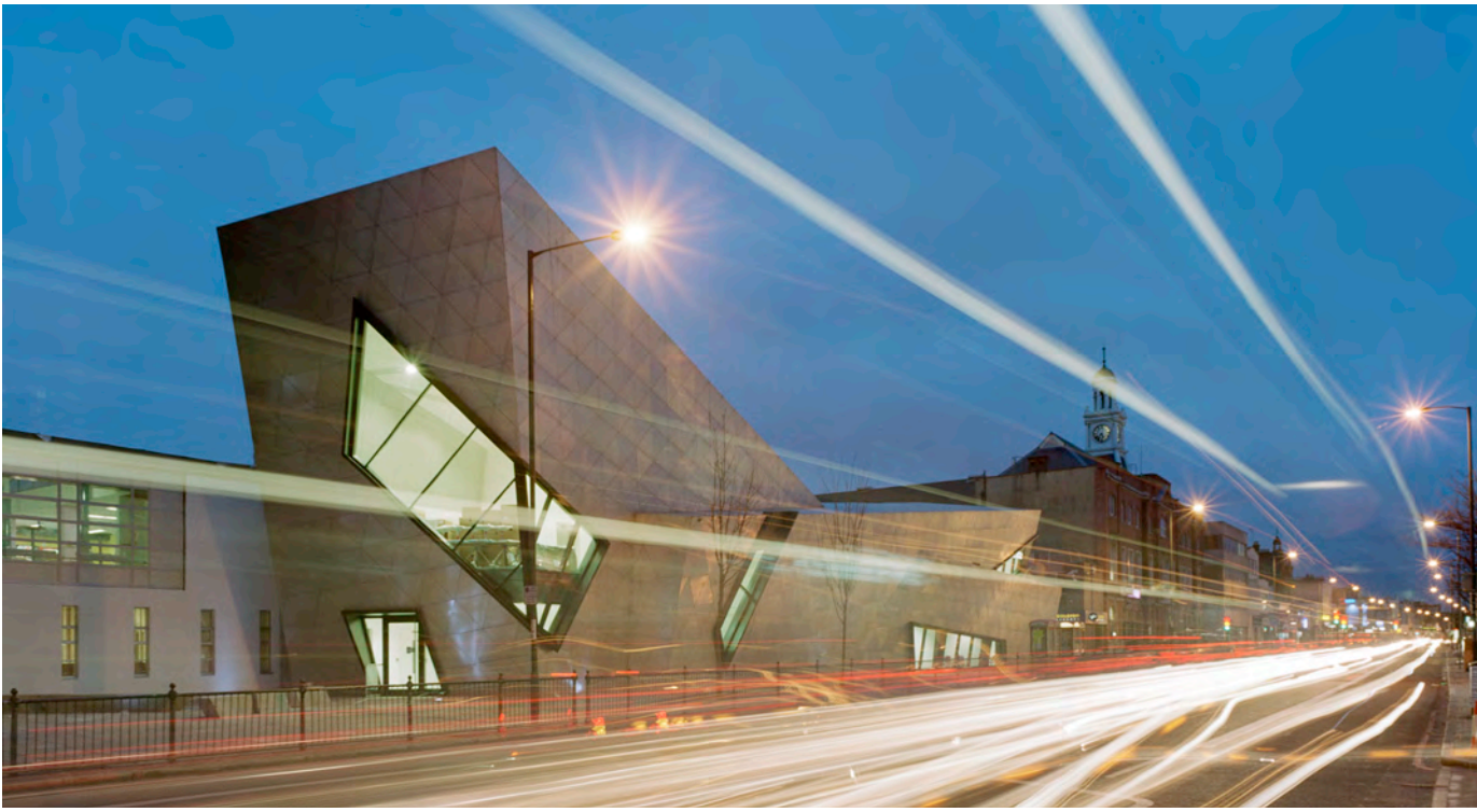
Elevation from Northeast
