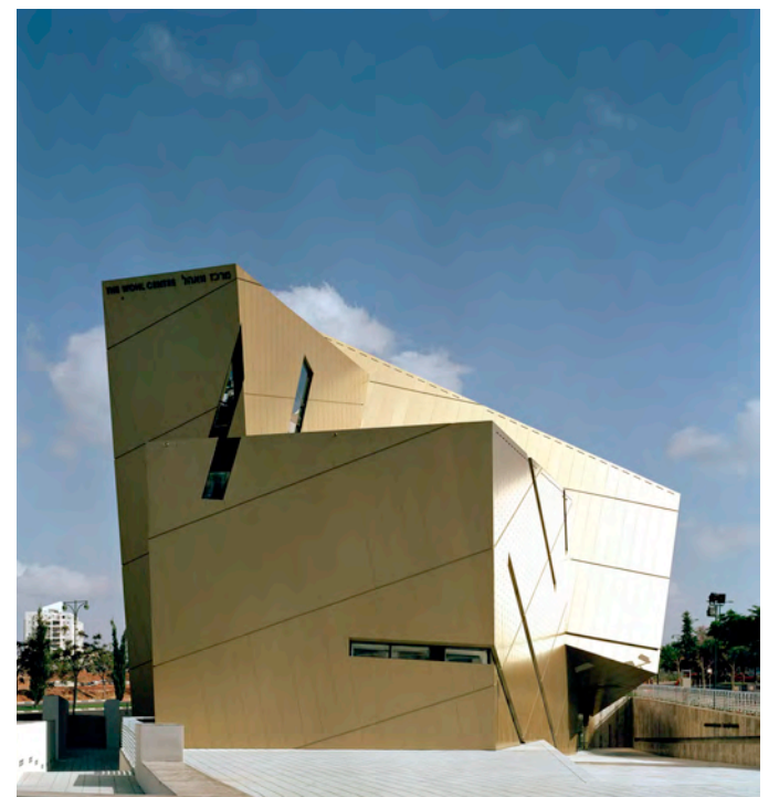
View of West Elevation
